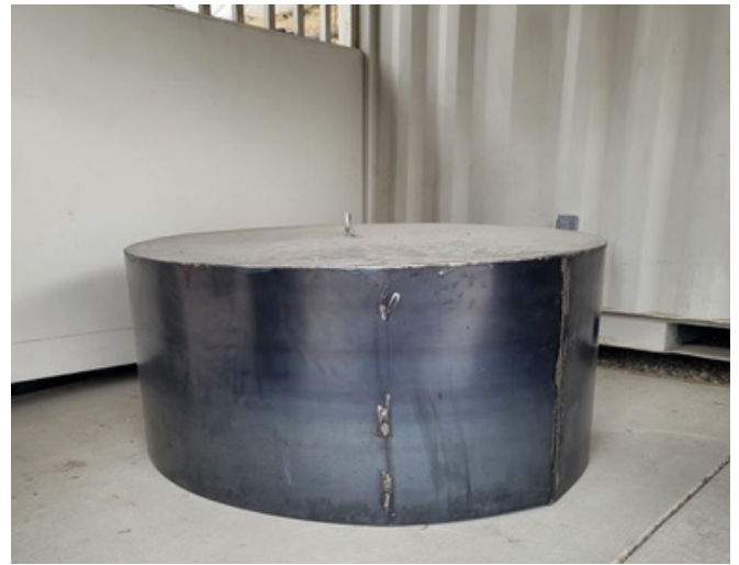
Newly constructed base for the water jacket
